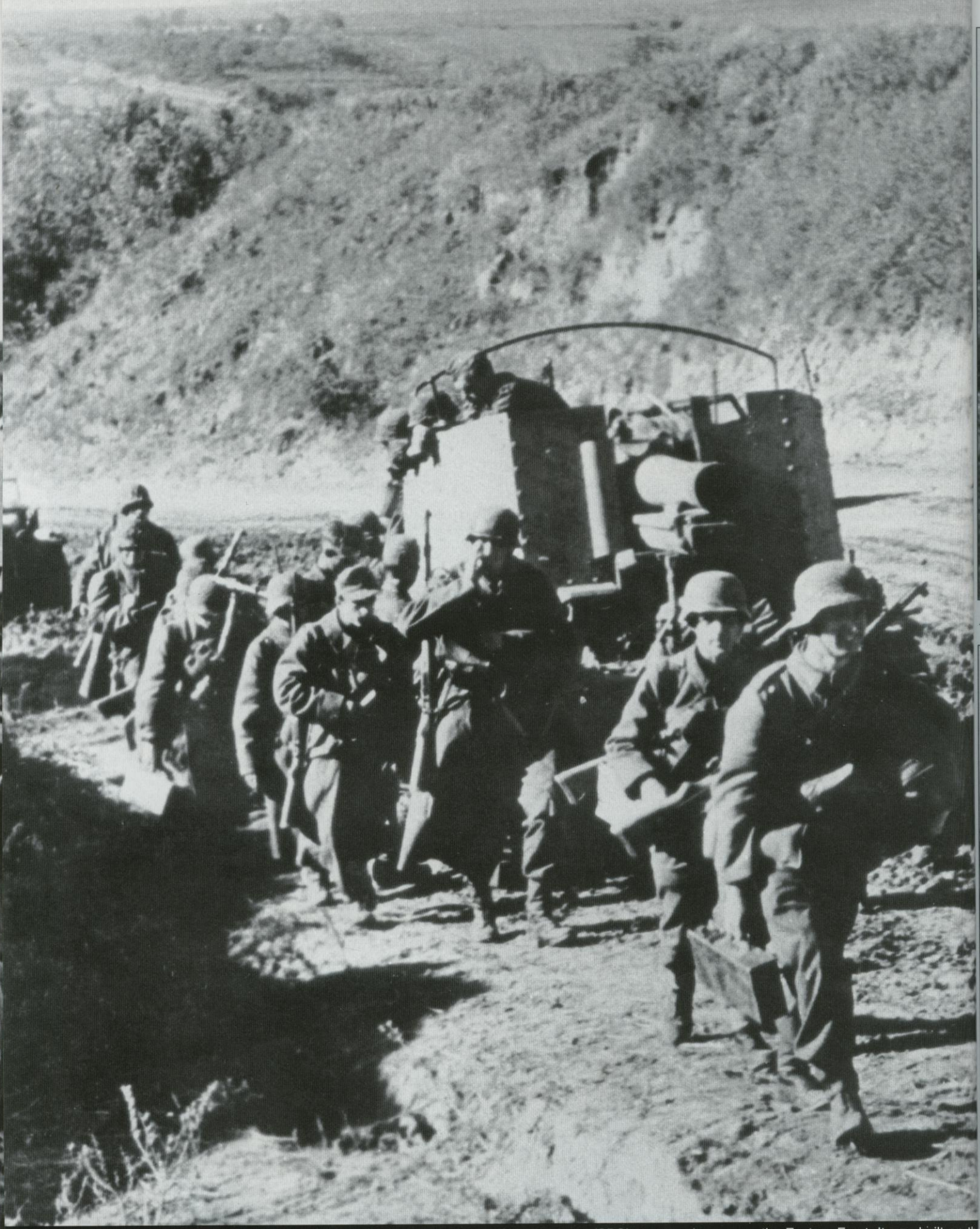
The vehicle shown here, the Sd.Kfz. 138/1 Grille (cricket) heavy self-propelled gun (SPG), was rarely seen on the Eastern Front. It was built on the Pz.Kpfw. 38(t) chassis and was armed with a 15cm sIG 33 gun. About 100 of these vehicles were produced between the beginning and autumn of 1943. They were used in the artillery units of infantry regiments in Panzer divisions.
