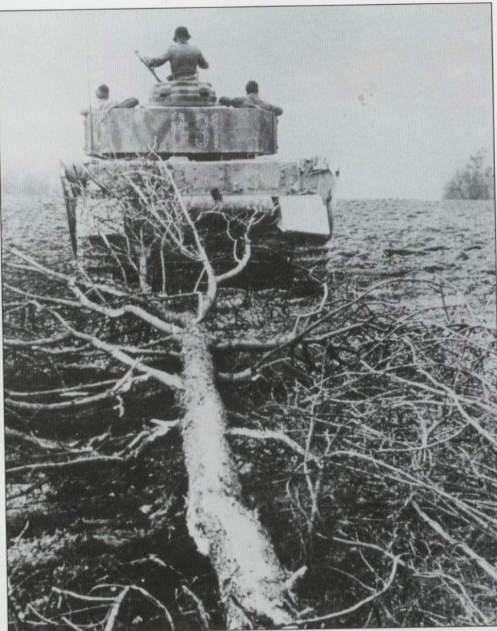
The crew members of a Pz.Kpfw. IV Ausf. H demonstrate that a tree is no obstacle for a German tank. This photo shows to advantage the system of installing side skirts on the superstructure. The tactical number is painted in the standard way — the first figure, which indicates the 8th company, is separated from the two others, which indicate the 1st tank in the 3rd platoon, the vehicle was used by the platoon commander.
