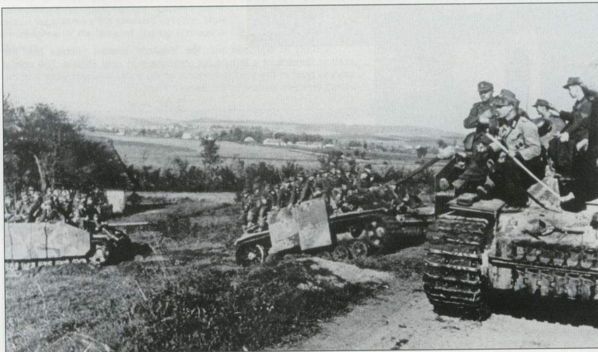
A group of soldiers awaits orders next to a Sd.Kfz. 250/3 leicht Funkpanzerwagen ground-to-air communications post, which is equipped with a frame antenna for the FuG8. The armored shield for a machine gun installed in the rear position is quite an unusual modernization.
